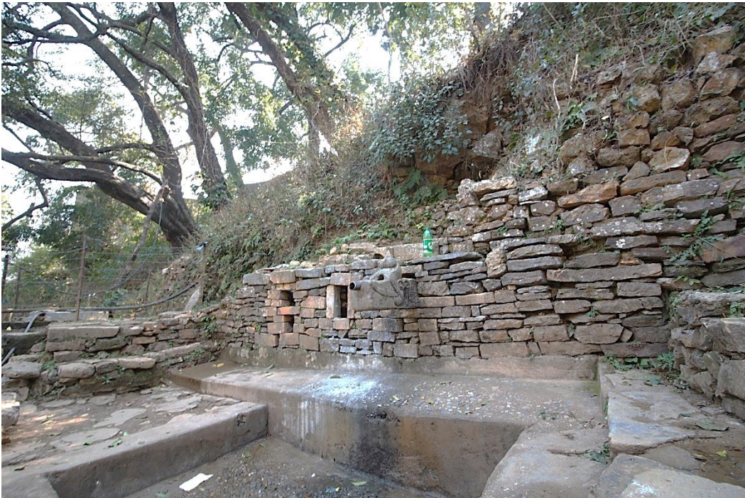
Photo 2: An Almost Dry Stone Spout
