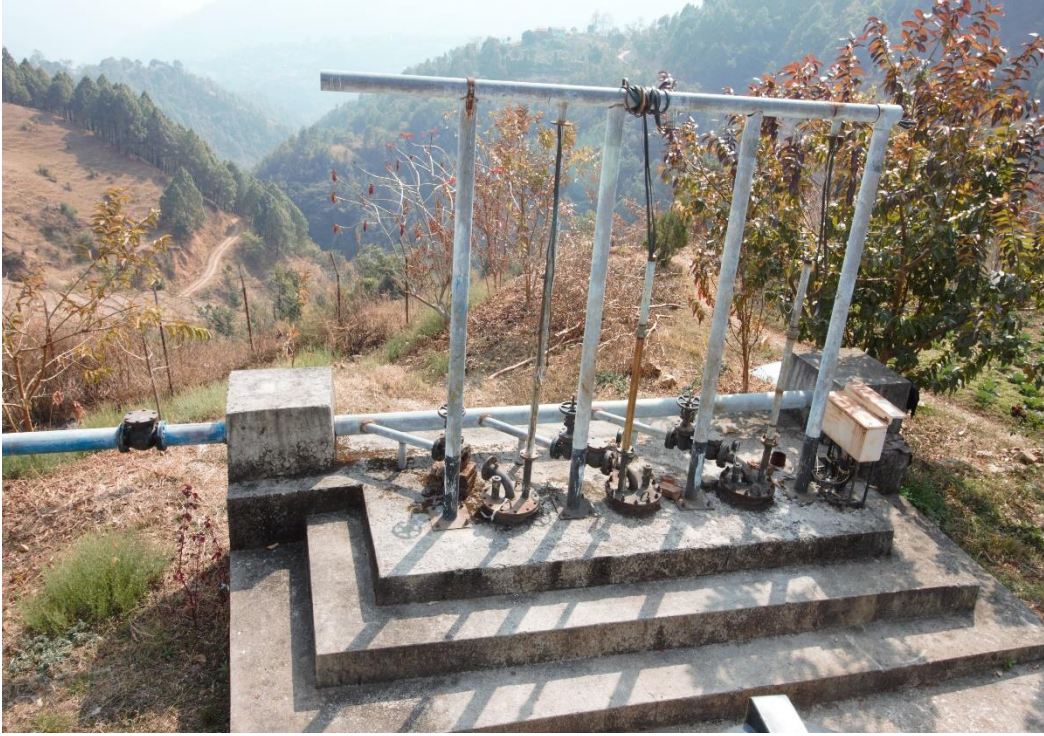
Photo 5: Infrastructure of Sisne Water Supply System
