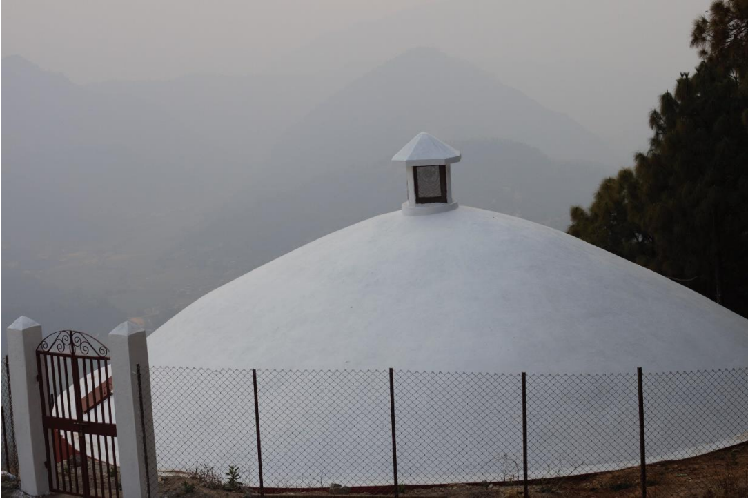
Photo 13: New Storage Tank under Construction
