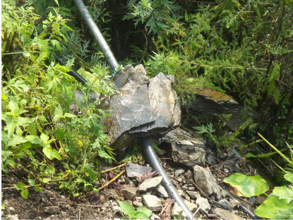
PLATE 4.5: Pipe connectivity from source (Khani Khola) to the village (Photo- Rashmita Sarkar, April, 2016)
