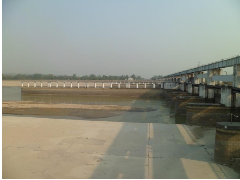
Photograph 11: Gandak barrage at Indo-Nepal border near Tribeni
