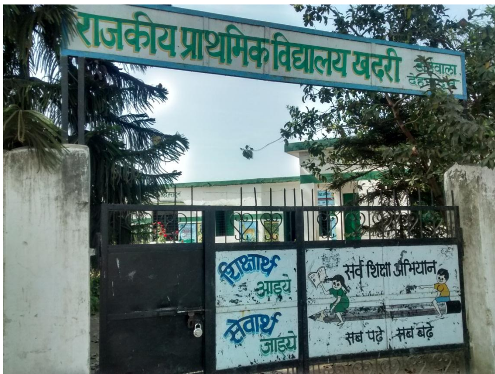
Primary School in Khadri Khadak Maf
