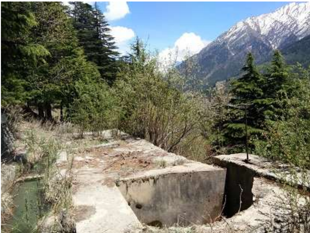
Picture 2 Growth of plants and grass on forebay tank of Harsil MHP
