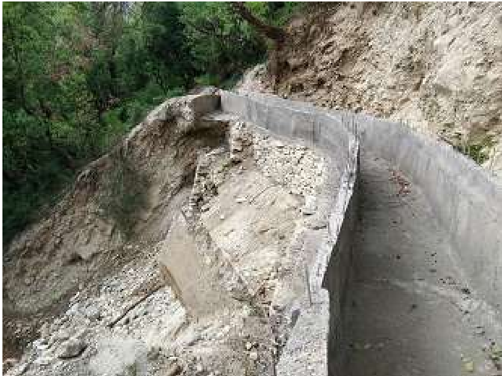
Picture 6 Reconstructed power channel of Gualri MHP
